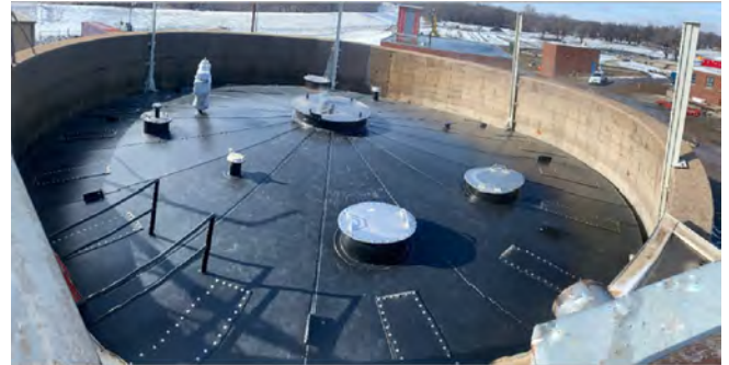
Gasholder Beam Digester Cover
